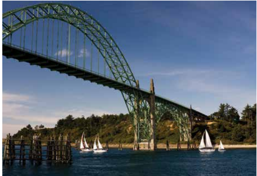
Sailing commonly takes advantage of protected baywaters.
