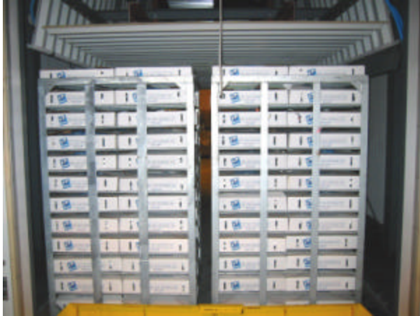
Figure 1. Blast air in the original (unbaffled) cell flows from right-to-left; air by-passes over the top and around the near and far ends.
