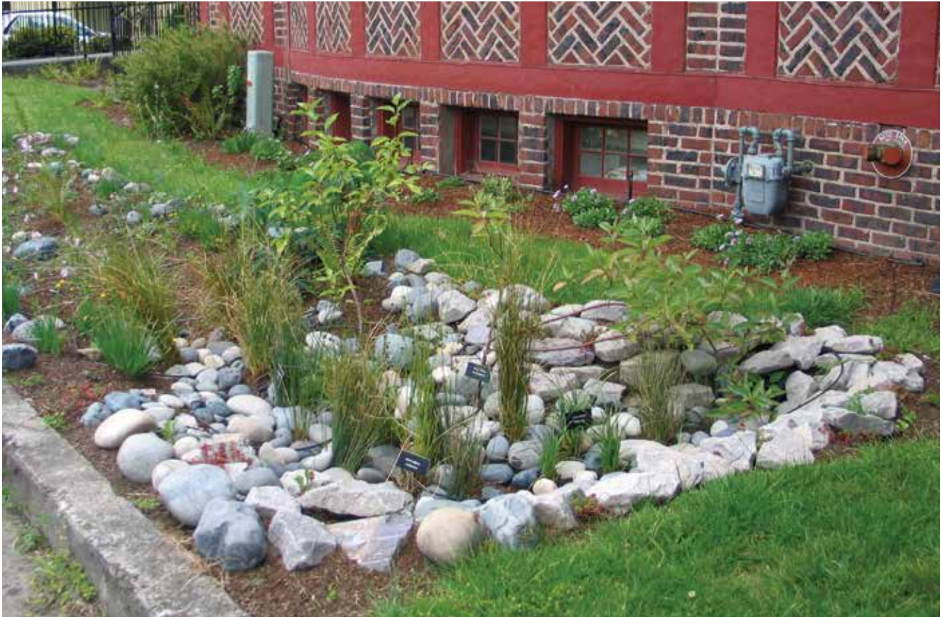
A newly established rain garden in Gresham, Oregon.
