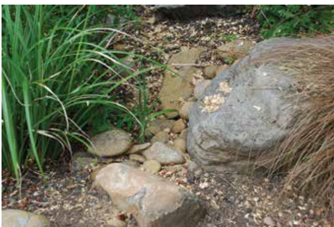
An outflow notch in a Portland, Oregon, rain garden, protected by rock to prevent soil erosion.
