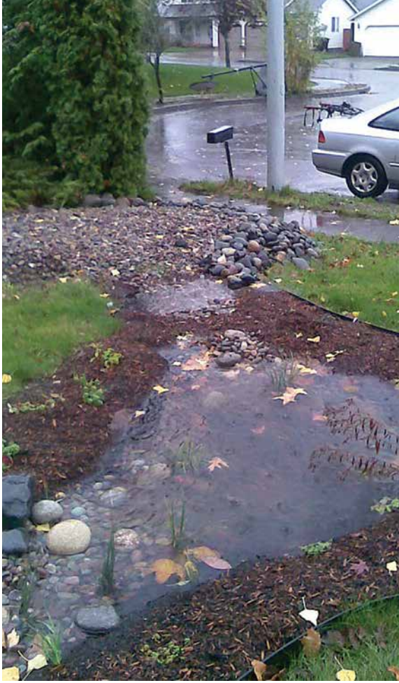
A rain garden in Gresham, Oregon, fills with rain. Note the use of rocks at the outflow point near the top.
